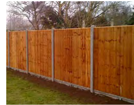
Timber Panel & Concrete Post in rear gardens
