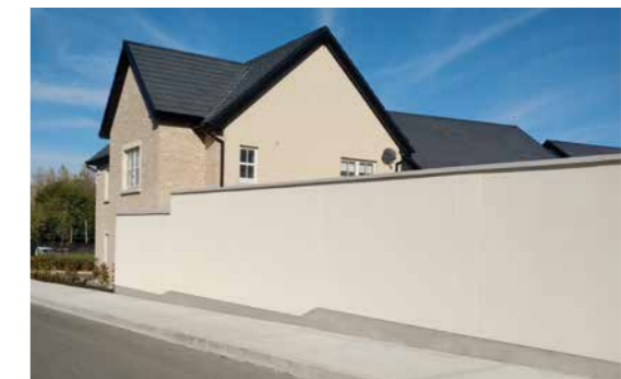
Rendered Concrete Block Wall with PC Concrete Capping to public realm areas
